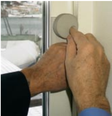
Fig 3. Drilling with the Coating Drill on a window-frame
